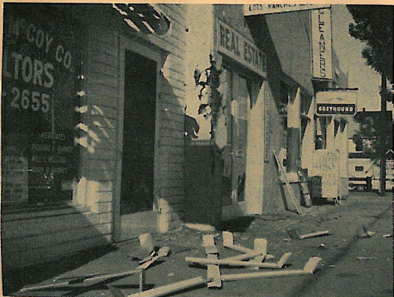
View of the damage to the awning and stucco on the George Butcher Building on Highway 80, Alpine, caused by truck wheels. Echo Photo.
